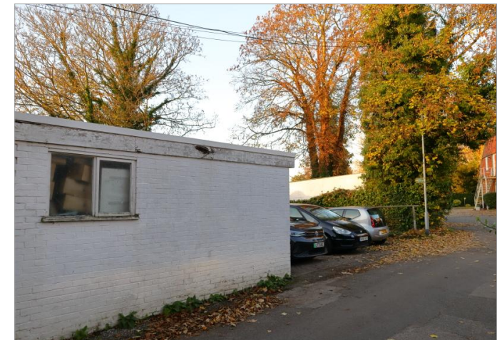
Garage and public footpath from South
